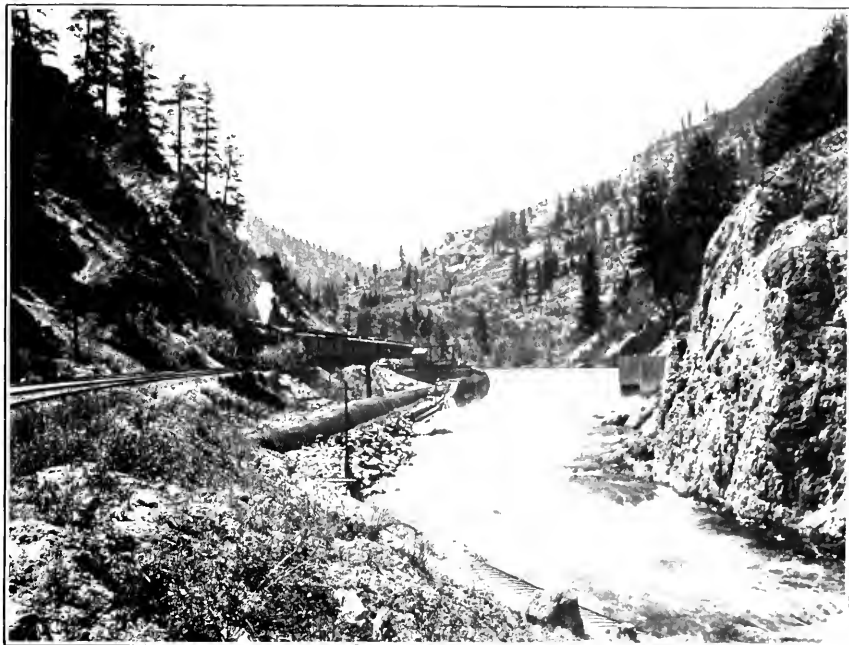
1. TRUCKEE RIVER CANYON NEAR FLORISTON, CAL.
